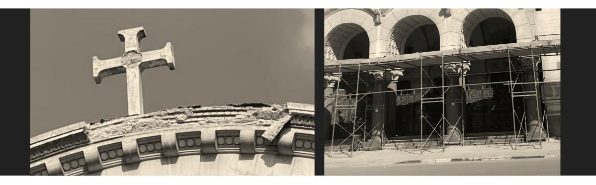
We knew we needed to act fast when a **dangerous incident** occurred on **October 15th, 2021** at 5:00 am, the stone medallion attached to the **roof cross broke and fell to the ground**, causing damage to the corniche underneath it and endangering pedestrians. We knew then that it was time to repair and preserve our beloved church. We installed scaffolding and are now only using the main entrance on rare occasions to ensure the safety of our people.
